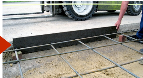
Joint filler at isolation joint (WR Meadows)
