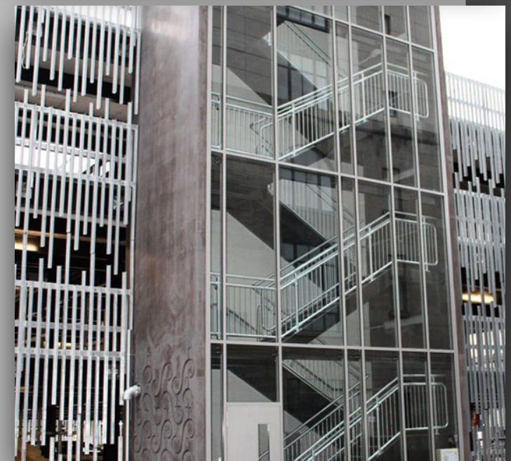
Pre-manufactured stairs and curtain walls are “delegated design” items.
